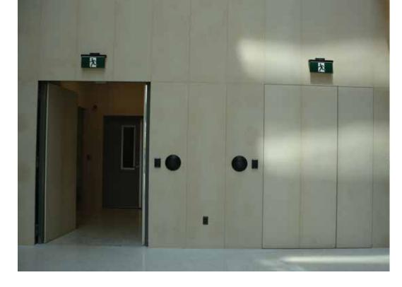
These acoustic door assemblies are slate-clad, designed to integrate with existing slate walls and are installed flush with the surrounding façade.
