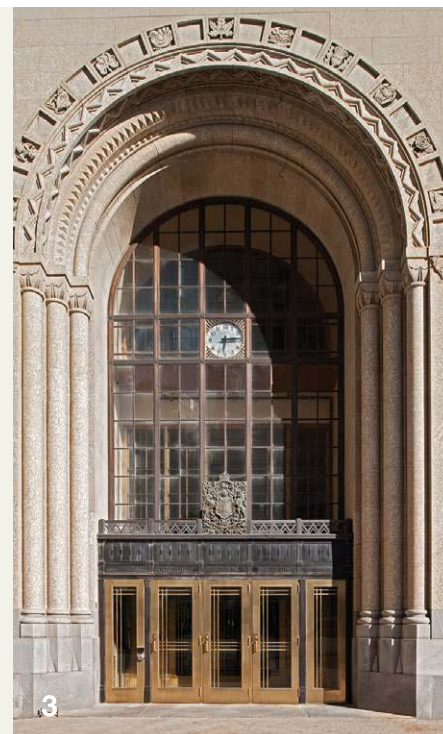
"After" view of the entire front façade, with doors replaced and bronze area above the doors cleaned and polished. Other items have been removed from the glass panels above the entryway.
