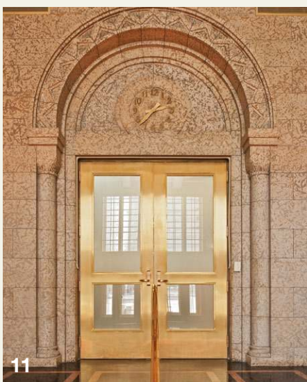
Bronze-clad double swing doors leading from the interior of the building into the main foyer and front entrance of the building
