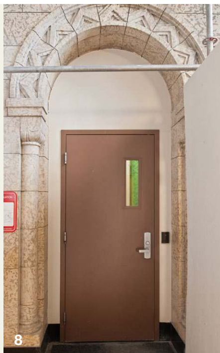
"Before" photograph of painted hollow metal door to stairwell
