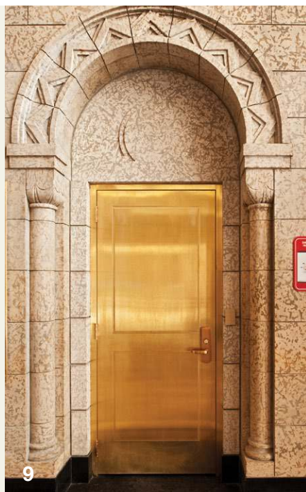
"After" photograph of door to stairwell, etched and fire-rated
