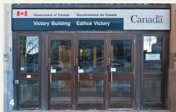
"Before" shot of the front entrance bank of doors, sidelites and frames clad in anodized aluminum from the 1960s retrofit
